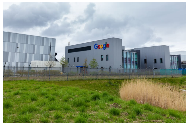
Google's data centres now use AI to reduce cooling energy by up to 40 per cent
