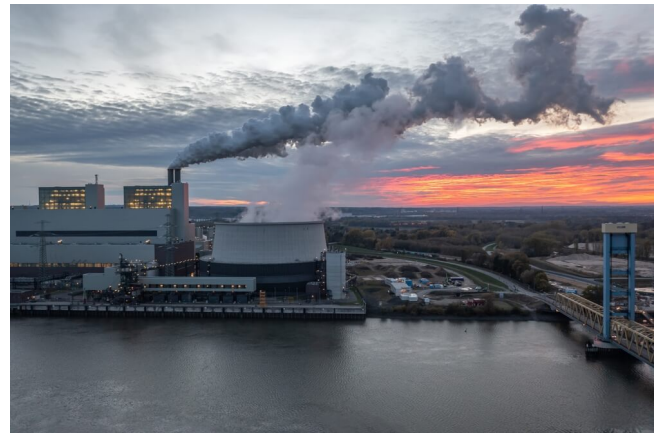
Moorburg power plant won a bid in the auction for the nationwide coal phase-out in 2020
